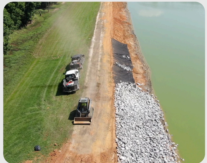
Repairs at the Philadelphia Wastewater Treatment Lagoon
